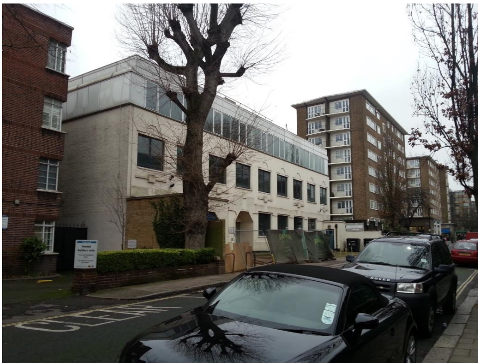
Prior to demolition views of the site from Wellington Road (top) and Cochrane Street(bottom).
