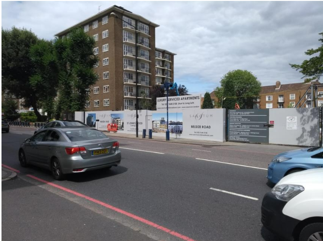
View of site from Wellington Road following demolition of the previous building pursuant to the February 2017 permission.
